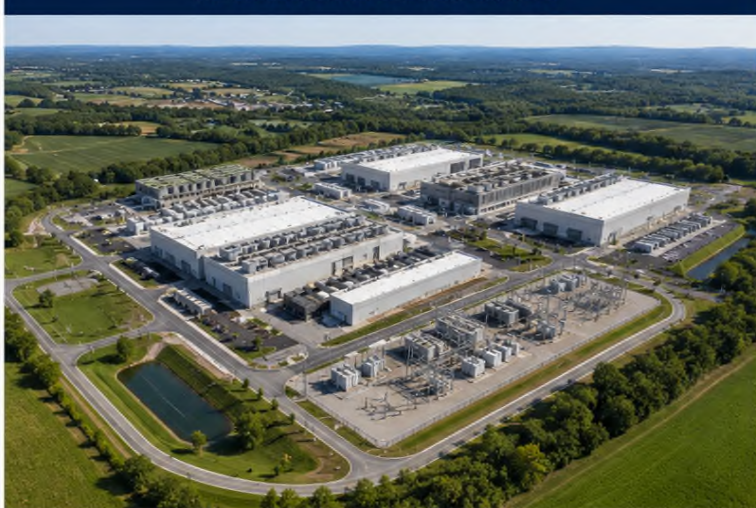
TYPICAL AI DATA CENTER CAMPUS
